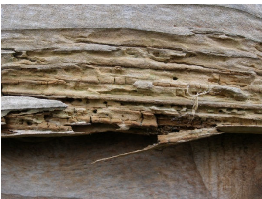
Image 0-4; Common furniture beetle damage
